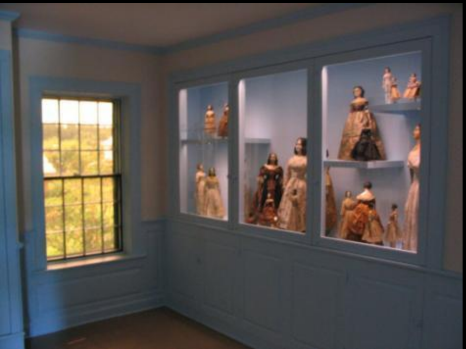
Bronze Tinted Plexiglas on Window 95% of Natural Light Blocked
